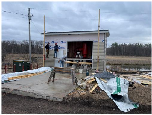
Photo #4: Continuing to nail on metal siding - Apr 23, 2024, 9:15 AM
