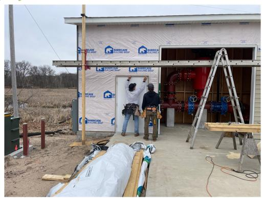
Photo #3: Nailing metal edging to the pump house around the service door - Apr 22, 2024, 1:02 PM
